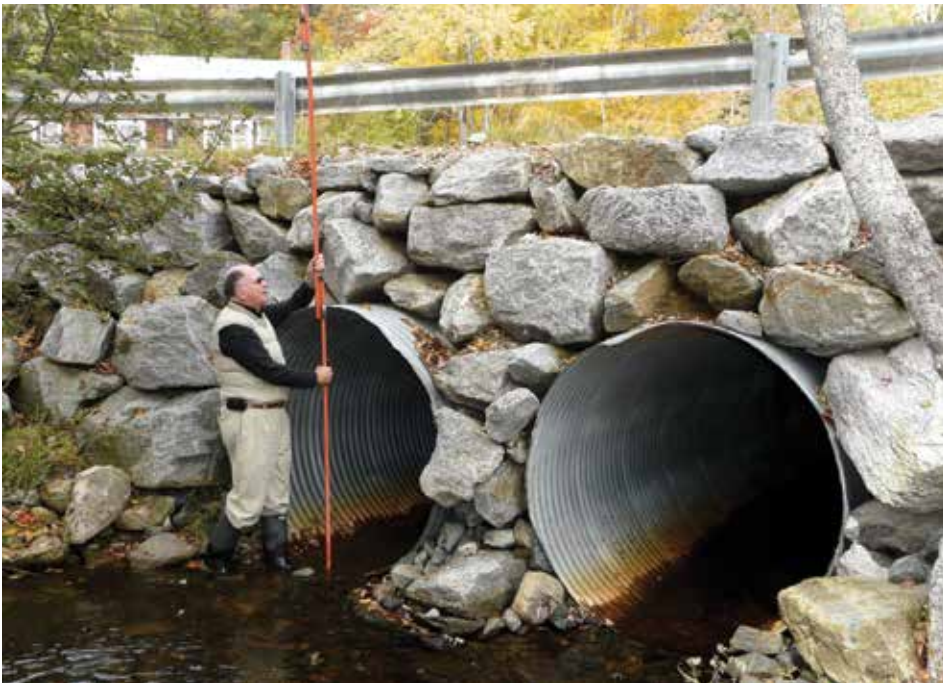
Figure 6. The LSPA responded to more frequent heavy rain events in the Lake Sunapee watershed by partnering with others to develop a climate adaptation plan focused on stormwater management, including recommendations for replacing undersized road culverts. Photo: Midge Eliassen.
